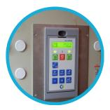
PUMPS Start and stop pumps via smartphone. In irrigation pipelines, raindancer® automatically switches the pumps on and off. If you have a frequency controlled pump, raindancer® can adjust the parameters dynamically.
